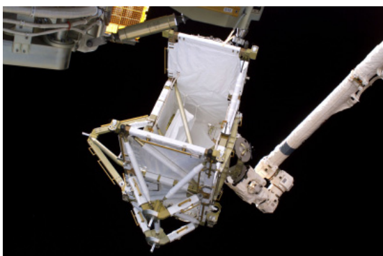
The new P5 truss awaits installation following the hand-off from the shuttle's robotic arm to the station's Canadarm2.
